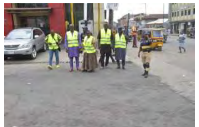
One of the completed road at Palm Avenue bus stop in Mushin
